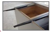
When used with overhangs less than 15", the IslandBar can be positioned further into the cabinet. Supports should be spaced no more than 16" to 20" apart for optimum performance.
